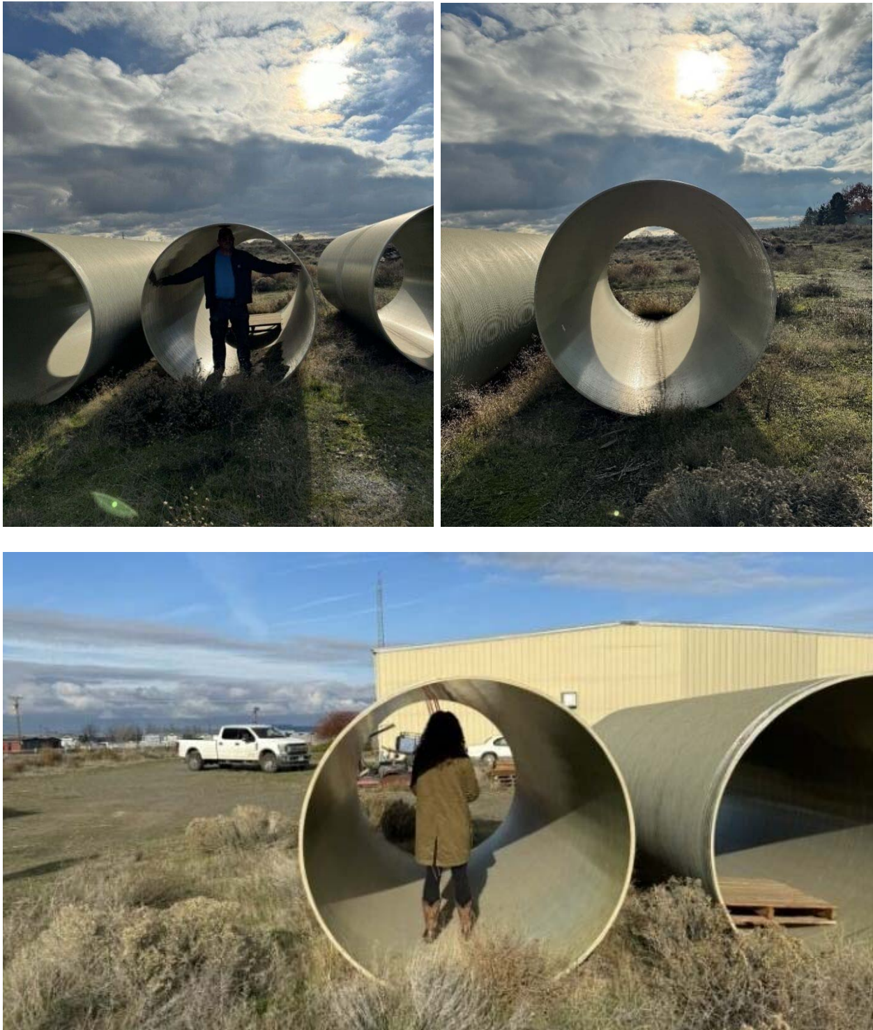
Images 3, 4, 5. Pipes used by the Port to transport nitrogen-rich wastewater to local farms. 2
